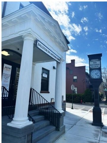
Ballston Spa National Bank’s renovated original home office at 87 Front Street in Ballston Spa. BSNB is the oldest bank serving Saratoga County.
